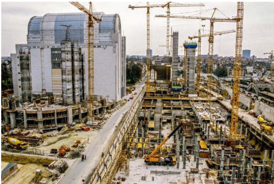
Construction works at the EP buildings in Brussels.
